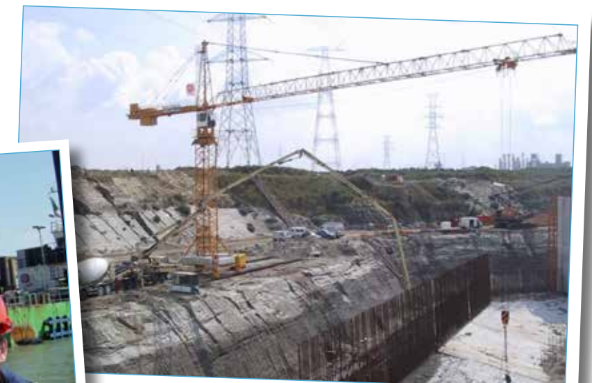
Construction works for the Deurganck dock, Antwerp
